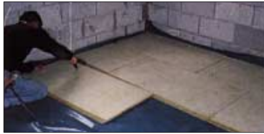
Rockfloor being laid
