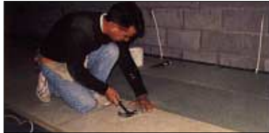
Chipboard being applied as a floating floor construction
