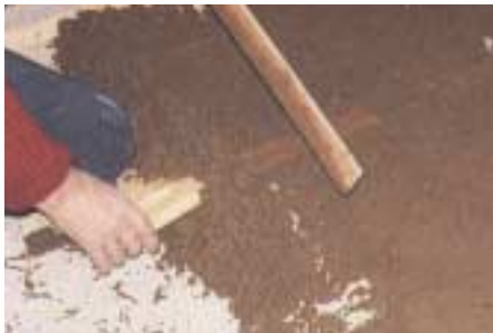
Applying levelling screed
