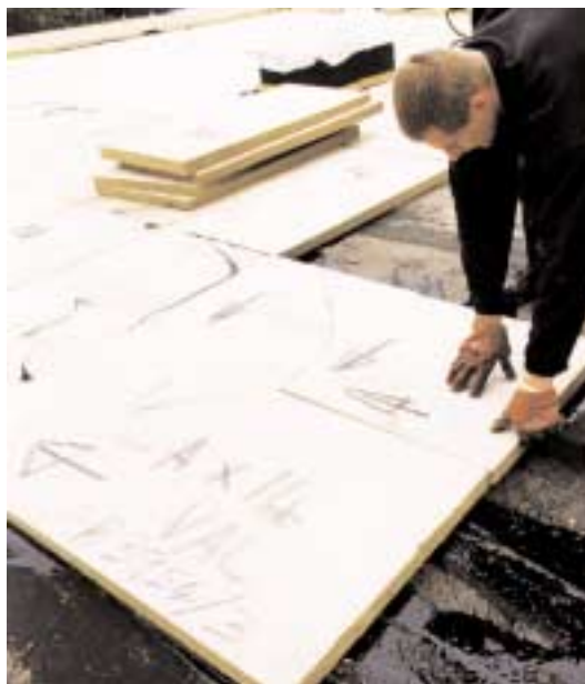
Typical application of pre-cut mitre
