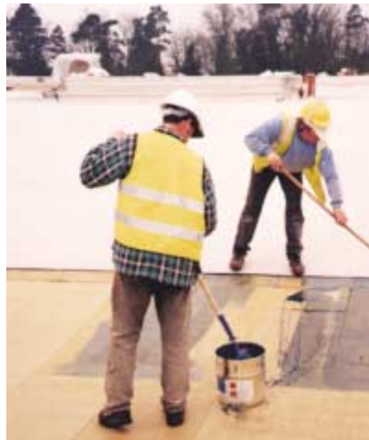
Application of adhesive to Hardrock Single Ply Adhered boards.
