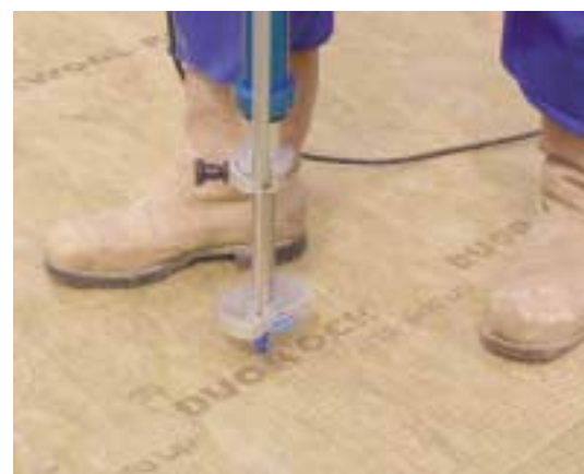
Application of a plastic tube fastener
