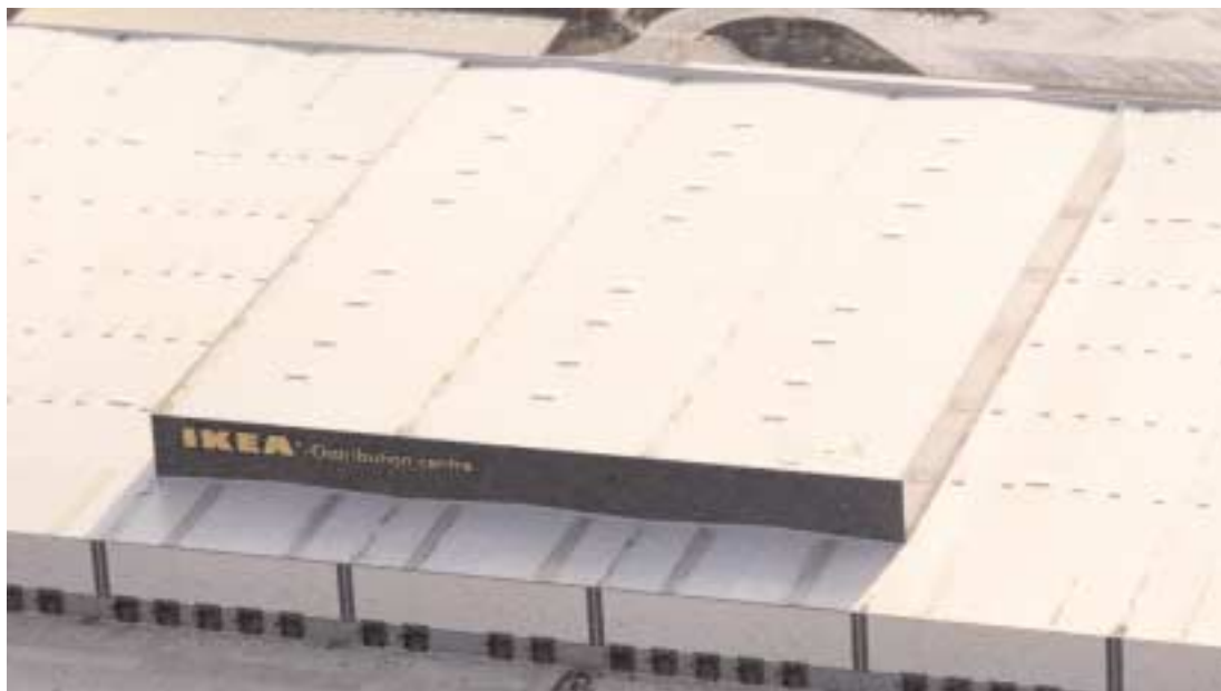
Right: Ikea distribution centre, Doncaster. DuoRock (Plain) Roofing Board, 60,000 m 2
