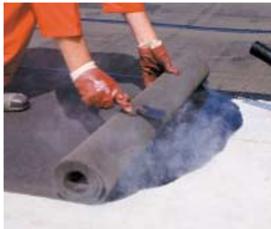
Typical pour & roll application over DuoRock (Tissue faced) Roofing Boards.
