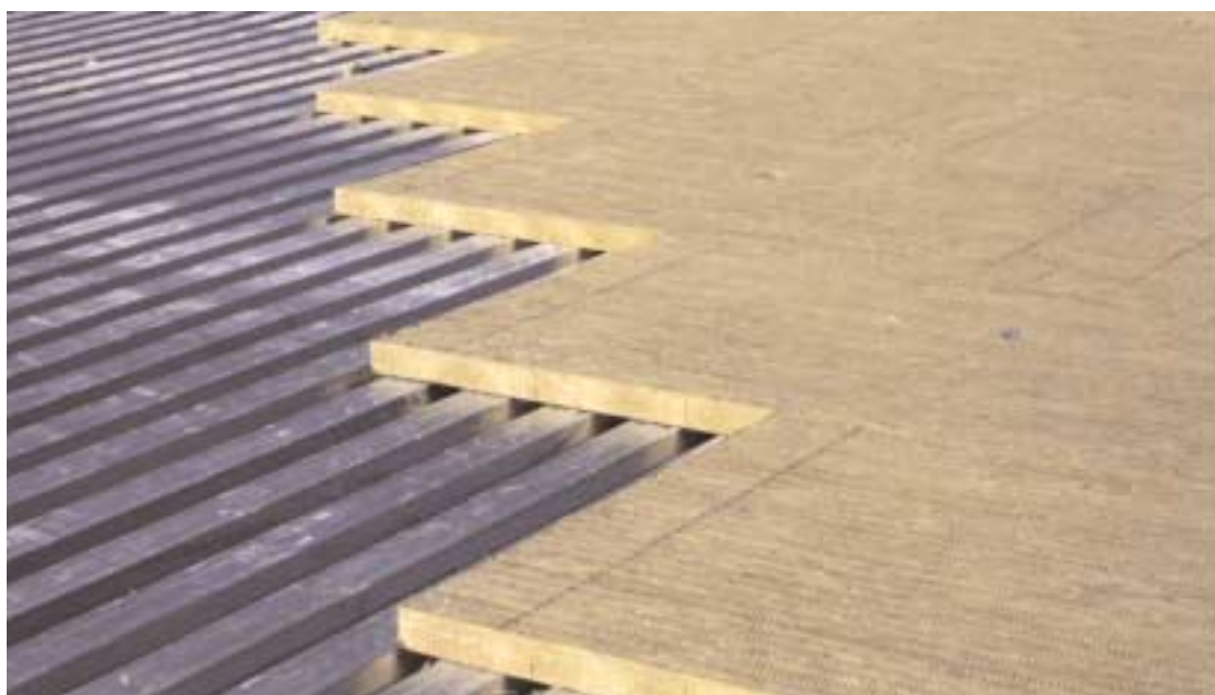
Right: Extension to factory, DuoRock (plain) roofing board.
