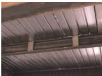
Noggings glued between steelwork flanges
