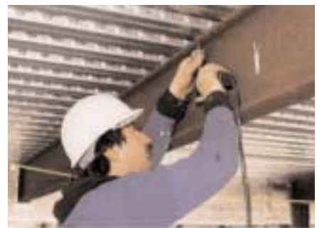
Fixing stud welded pins
